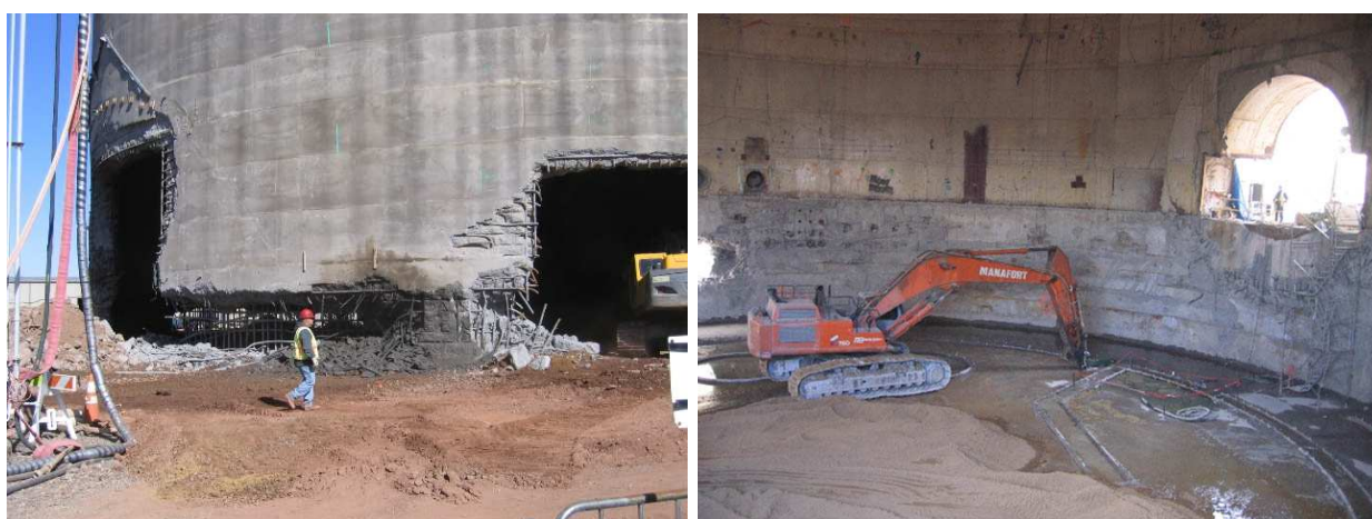
Obr. 6: Demolice kontejneru JE Connecticut Yankee ( http://www.world-nuclear.org/ )
